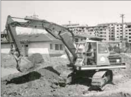
1976: S 517 with crawler chassis and plastic cab moving earth
