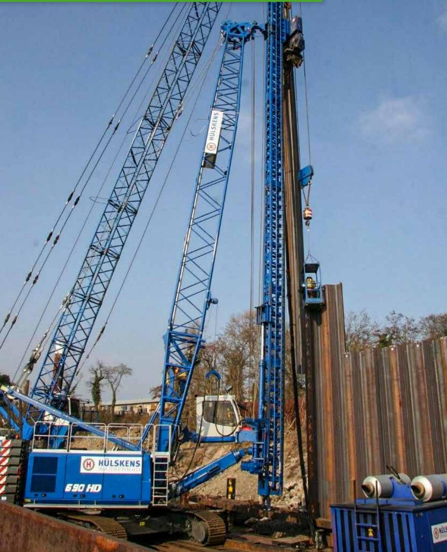
690 HD - Sheet piling, with leader in hydro construction; Germany
