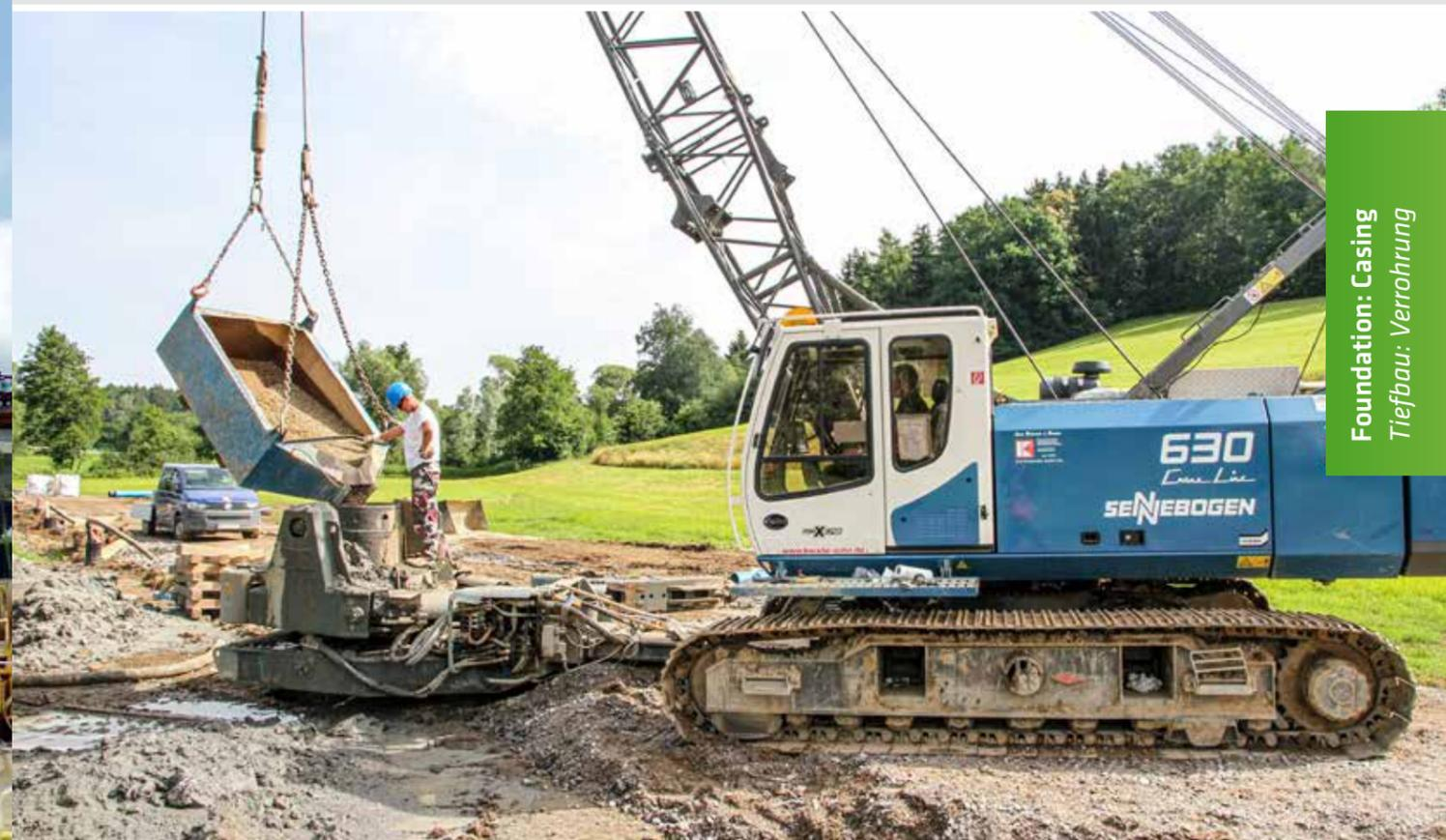
630 HD – Well digging with casing oscillator; Germany
