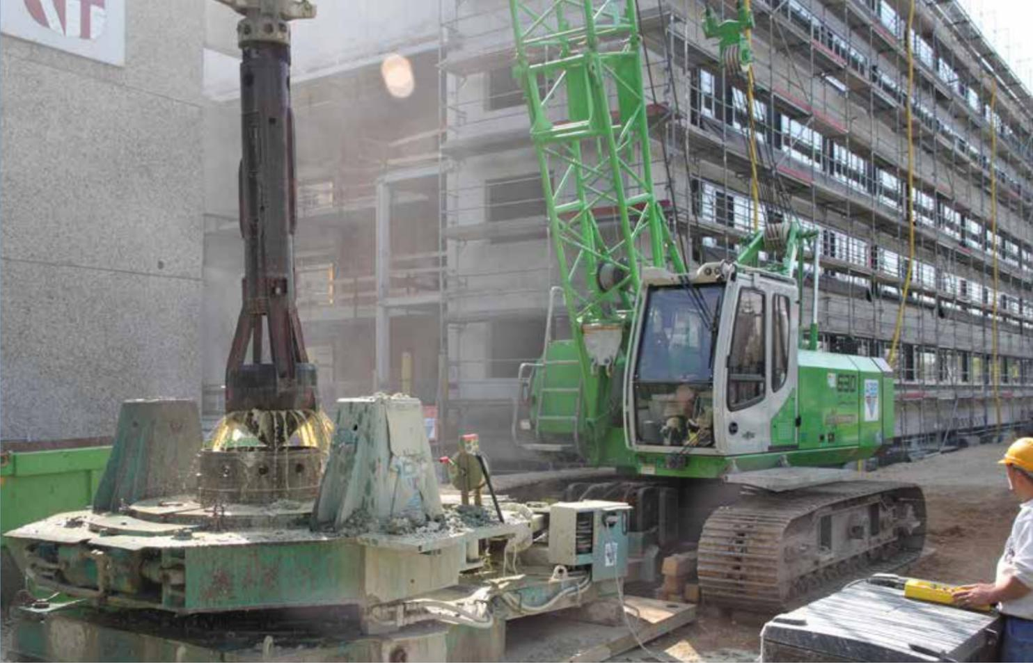
630 HD – Well digging with casing oscillator; Germany
